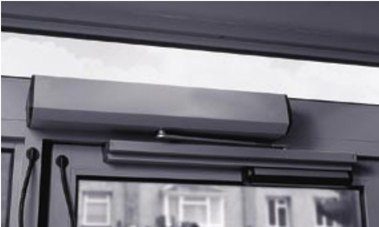
Above; Briton 2500 low energy operator
